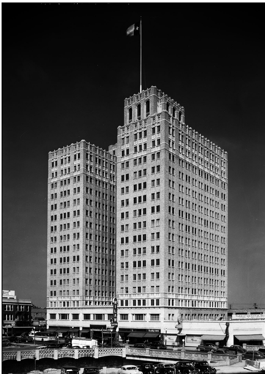
The Milam Building in downtown San Antonio, Texas. When completed in 1928, it was the first fully air-conditioned high rise office building in the world. The press at the time praised the AC fabricator and supplier Carrier Corporation for being able to "manufacture weather" and "make every day a good day" inside the building.
